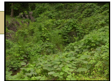
"Before" shot of a culvert overgrown with kudzu, and posing a hazard for Norcross streets.
